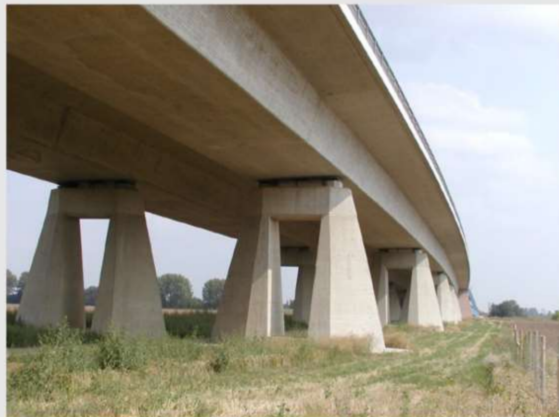
Saale River Bridge at Beesedau. Part of motorway A 14
